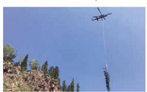
Tree removal by helicopter is the only practical method of vegetation clearing in the high mountain terrain. By law, wherever a helicopter bearing load will cross the highway, the road must be closed.
